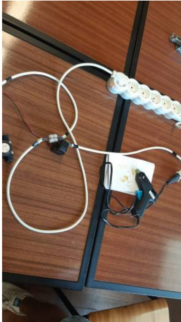
Figure 53: Photo of the real electronic of the project
